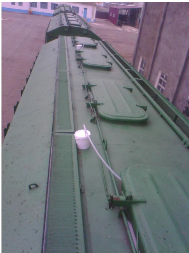
Fig. 2- Application of SGF-M2 generators to a hopper car through loading hatches #1 and #3
